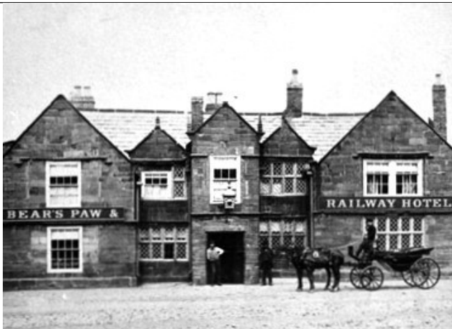
FDN2052 The Bear's Paw & Railway Hotel before early 20 th century restoration
